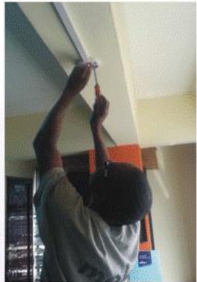
Our technical staff installing smoke detector
