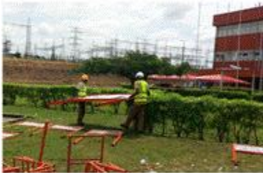
Our Project Team during installation of safety signs on site
